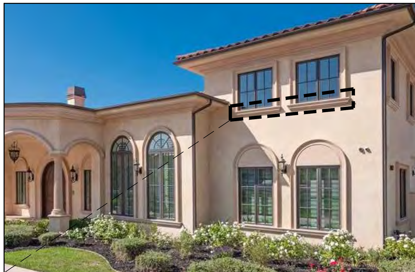
17. STUCCO OVER FOAM SCALLOPED SILL
