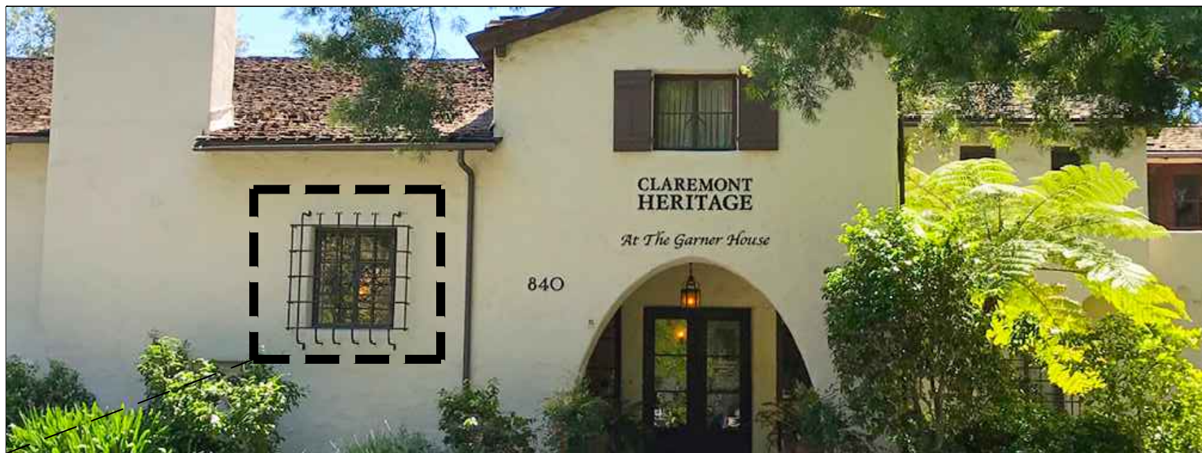
14. DECORATIVE METAL GRILLE WORK
