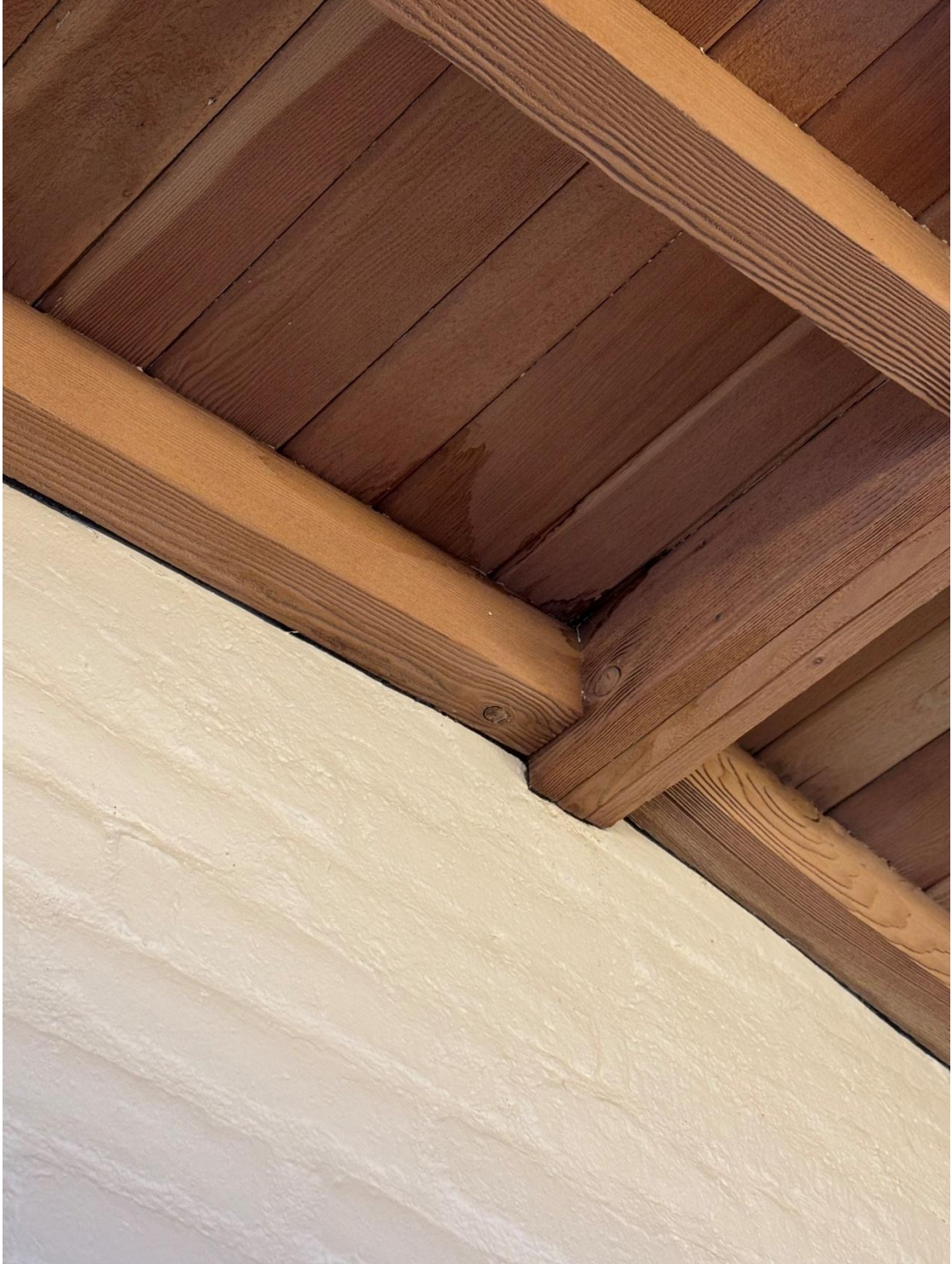
Roof Water Damage From Rain
